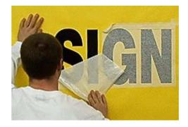
**Step 8.** Inspect the decal for air bubbles or wrinkles. Poke any trapped air with a pin and press with fingers. Stand back and your instullation is complete.
