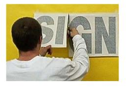
**Step 3.** Apply masking tape horizontally over the top edge of the lettering to serve as a hinge.
