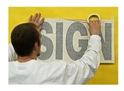
**Step 5.** Raise the lettering up over the top hinge and peel the liner back a few inches at a time.
