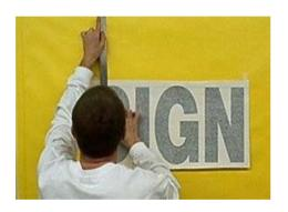
**Step 4.** Cut between each letter or number so that each is independently hinged from the top. (Skip this step and go to step 5 with small lettering or one piece decals)
